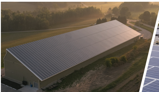
500kW Pitched Roof FIT 1
